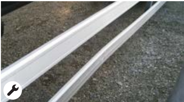
Bike racks: Deformation within economic repair
